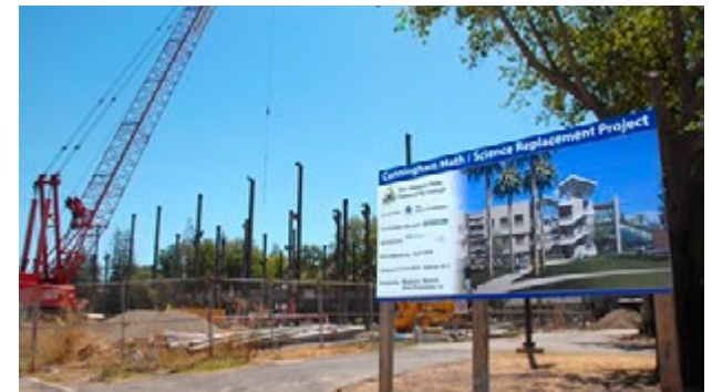
Construction of Delta's New Science and Mathematics Building
